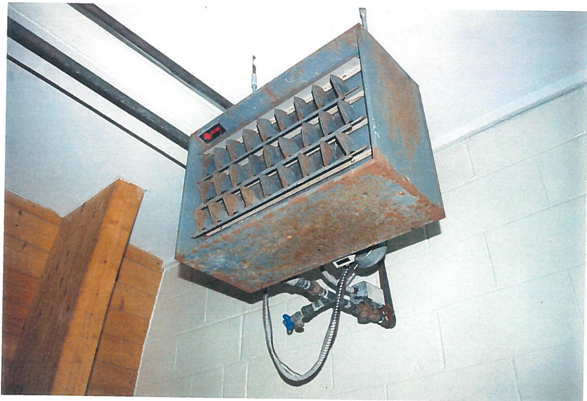
Existing corroded unit heater in locker room.. Ref. Section 2.6.1
