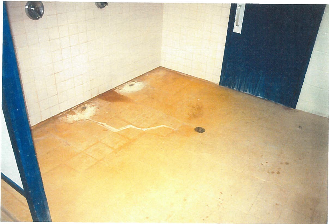
Miradur floor finish discolouration. Ref. Section 2.4.1
