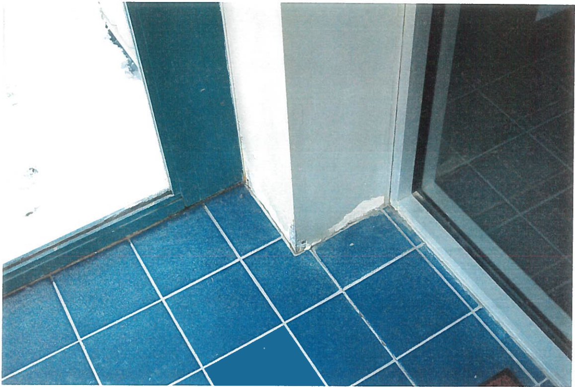
Tile base required. Ref. Section 2.4.2
