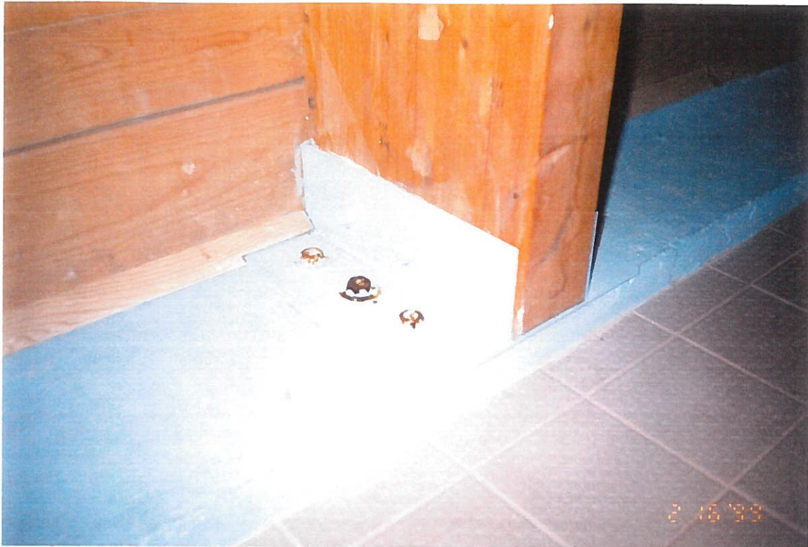
Glulam arch base plate. Note surface corrosion on anchor bolts. Ref. Section 2.2.4
