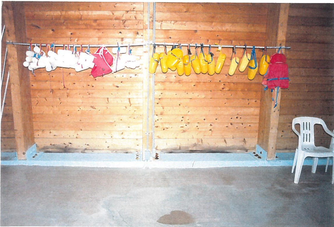
Wood wall finish deterioration and rust at steel fastenings. Ref. Section 2.4.2
