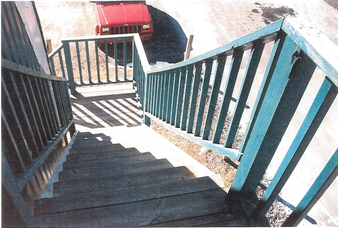
Stair and rails with excessively large openings. Ref. Section 2.3.5
