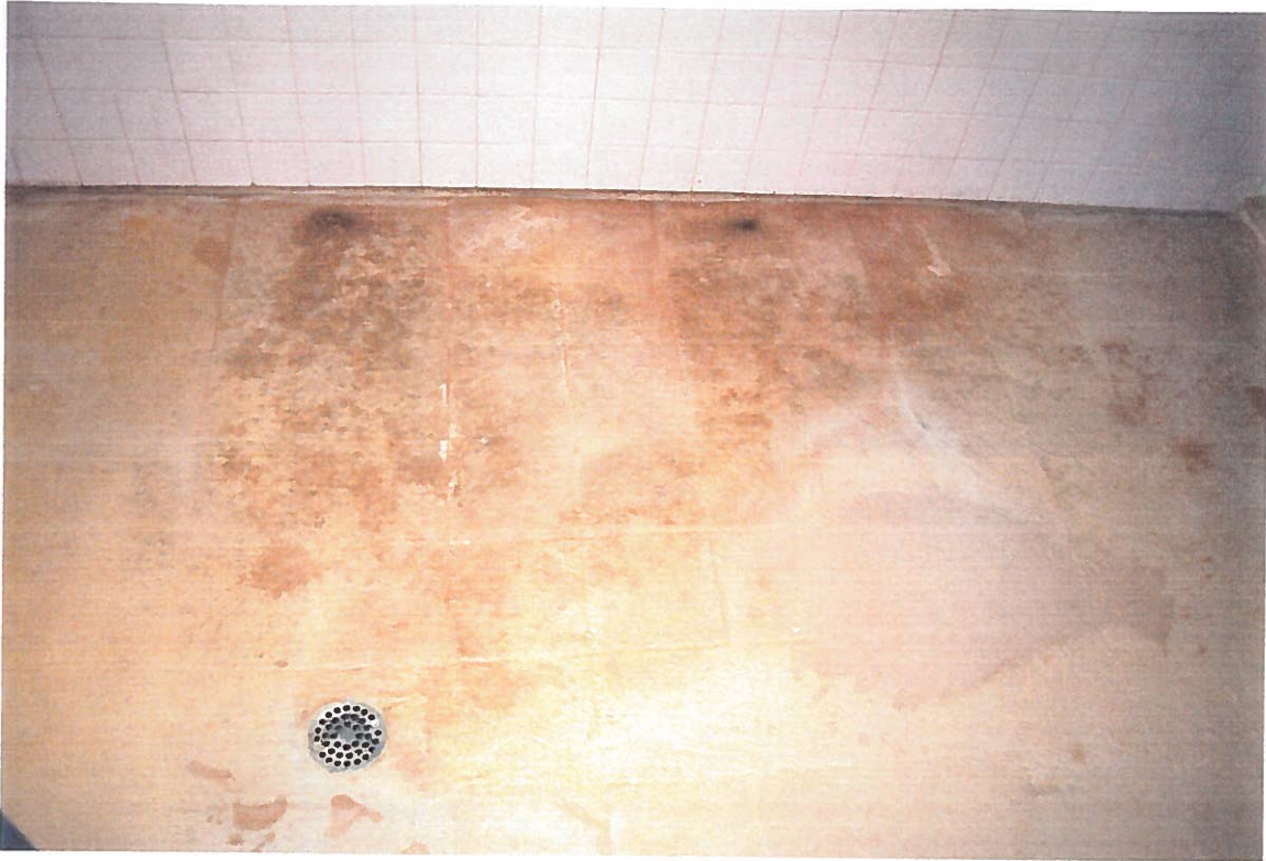
Miradur floor finish discolouration. Ref. Section 2.4.1
