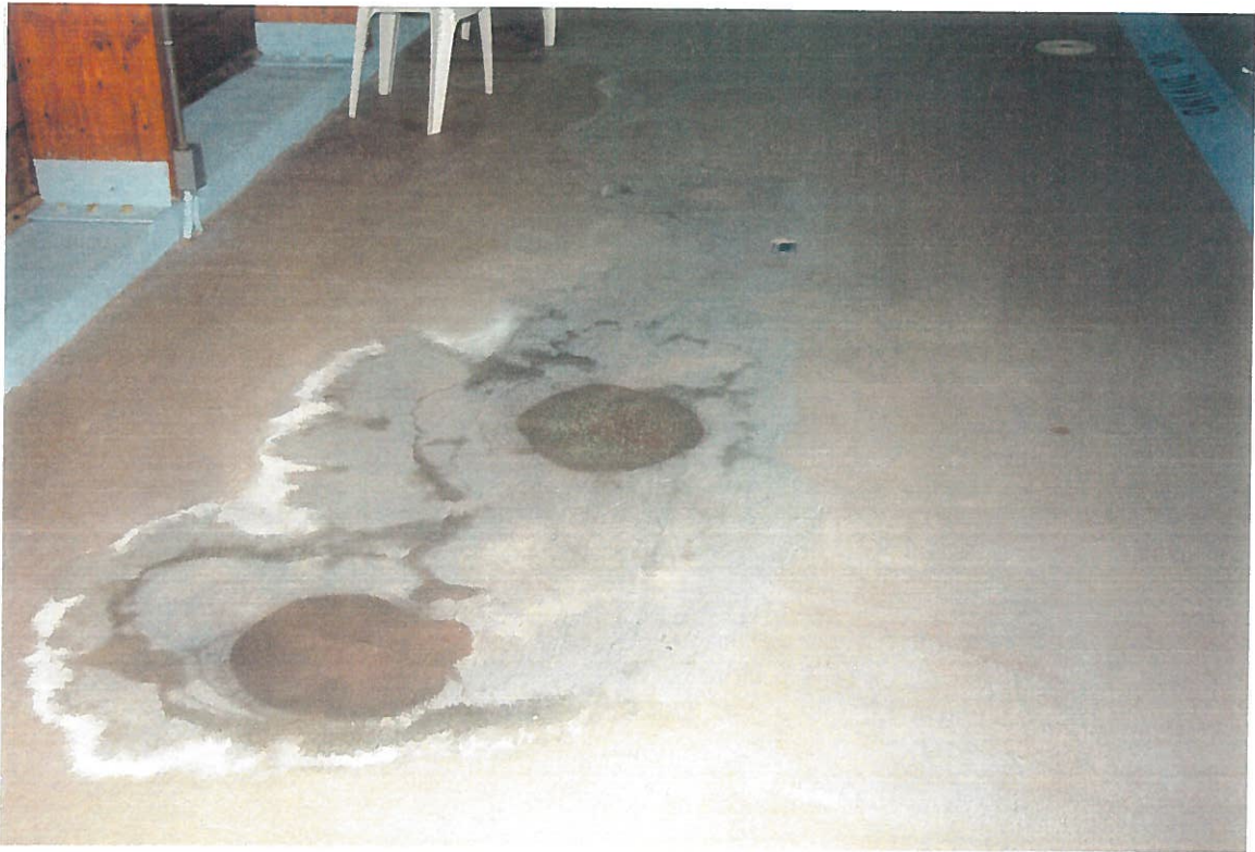
Miradur floor finish discolouration. Ref. Section 2.4.1
