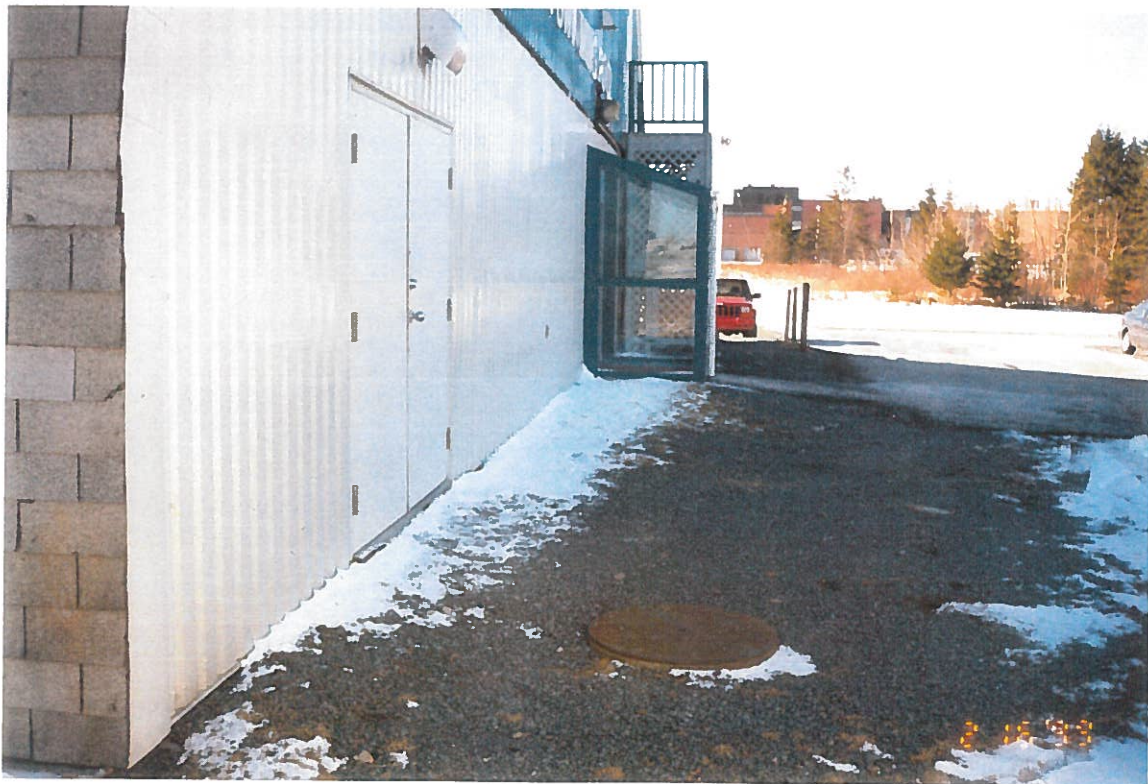
Excessive cross slope on paved area outside vestibule. Ref. Section 2.5
