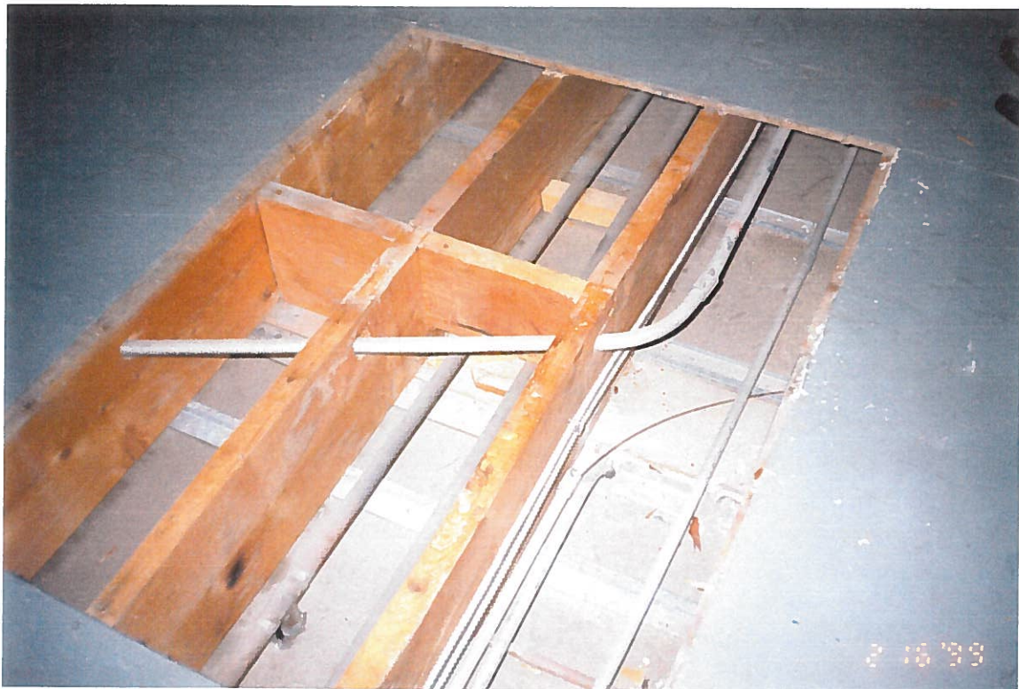
Plywood removed from mezzanine floor to view the framing for the mezzanine. Ref. Section 2.2.4
