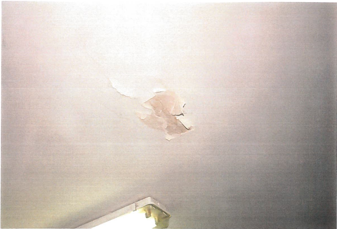
Water damage to ceiling at women's change room. Ref. Section 2.4.4
